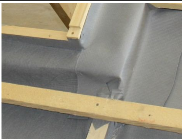
SKYLIGHT – detail of bottom corner
