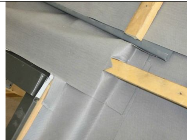
SKYLIGHT – detail of upper corner
